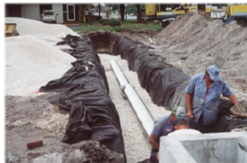
Underground Exfiltration Trenches
